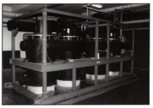
Each ORE-400 ice slurry unit consists of four ice generators. The units sit on top of the storage tank and drop ice slurry directly into the tank. A total of eight ORE-400 units (each capable of producing 500 tons of ice) are in the project for a total of 32 ice generators.
