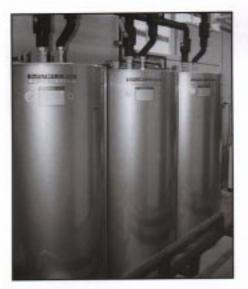
These Mueller tanks serve as hot water storage tanks. The hot water is produced by a Mueller refrigeration heat recovery system on the building's roof.
