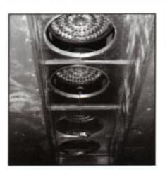
Photograph taken from inside the tank, looking up into an ORE-400 ice slurry generator. Each ORE-400 has a capacity of about 500 tons.
