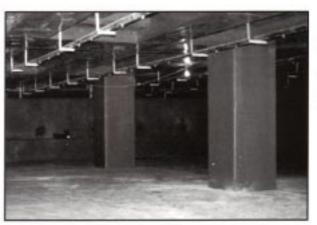
Inside the 36,000 ton-hour storage tank. Spray nozzles are shown along the top of the tank which will hold about 0.9 million gallons of 7% glycol solution.
