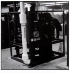
This is one of two 50-ton ice slurry generators installed at Mid-American Energy in 1996.
