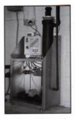
This 3-ton ice slurry generator and storage tank is used to cool the wort from about 210°F down to 46°F. A small 3-ton ice slurry generator can produce 504 ton-hours per week (3 tons x 24 hours x 7 days) for applications in process cooling and any short-duration load. These units have been installed in multiples for projects needing 6 tons or 9 tons of ice slurry.
