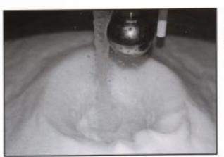
The ice slurry is pumped into the top of the storage tank. Note the spray ball which distributes the warm return solution over the ice.
