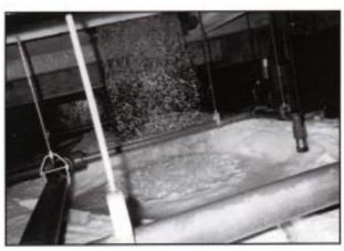
The ice slurry exiting a generator drops directly into the storage tank. If required, the ice slurry can be pumped to one or more tanks located remotely from the ice generator.
