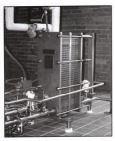
This **Mueller** plate heat exchanger receives cold solution from the ice tank to cool the wort.
